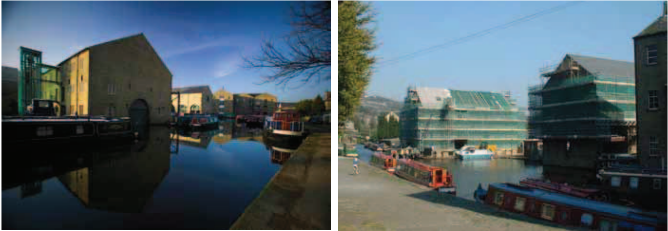
Regenerated No. 4 Warehouse, complete with wet dock and No. 4 and Salt Warehouses undergoing renovation
